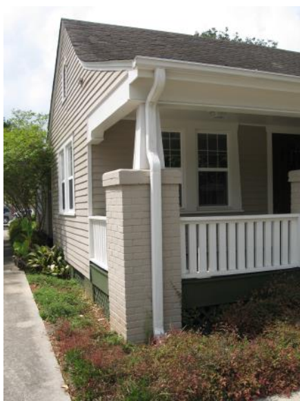
Appropriate design gutter and downspout at 510 Roussell Street.
