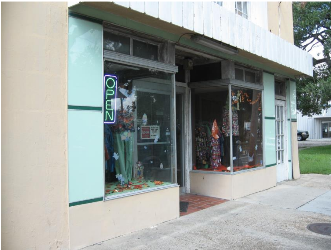
This original storefront at 244 Barrow Street possesses many typical elements: display windows, bulkheads, and transoms.
