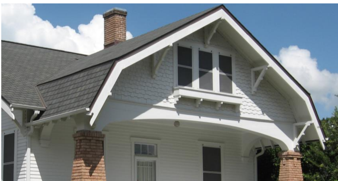
Exterior siding materials are also important in defining the style and character of a dwelling such as the wood shingles in the gable field at 631 Verret Street.
